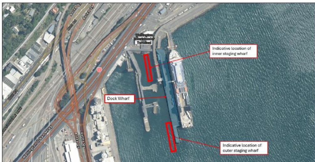
Figure 2. Existing terminal showing locations of staging wharves. Image from application.
