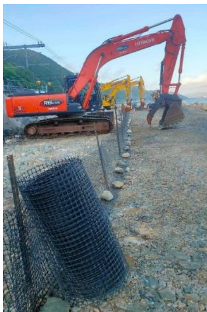
Figure 14: Examples of fencing to exclude kororā from work areas
